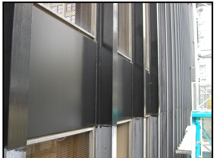
Freshly painted exterior surface
